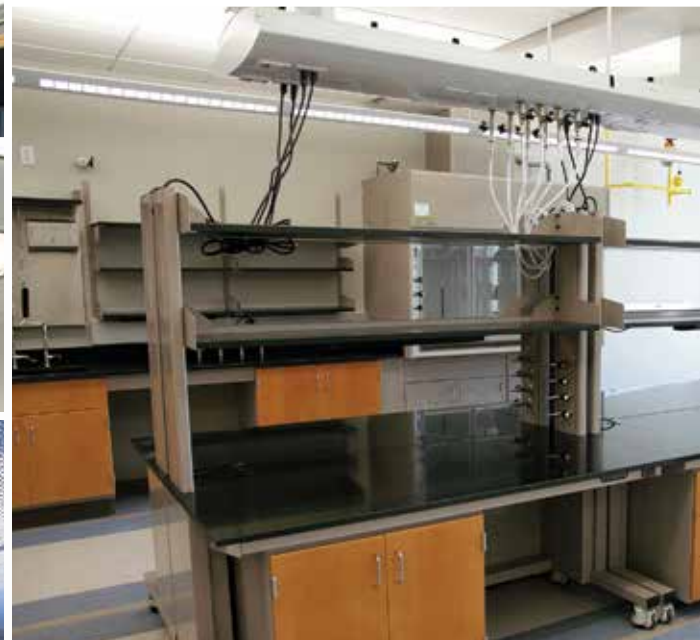
Overhead service enclosure with quick connect fittings
